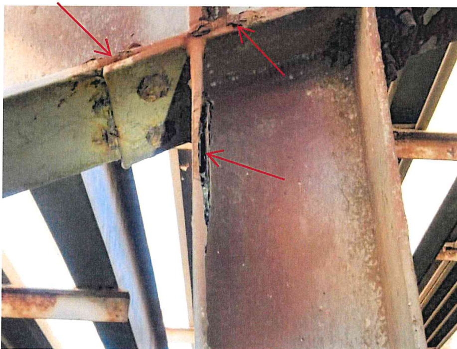
Figure 34 – Photo showing severe corrosion at column web & flange, column top plate, and steel beam flange (indicated by red arrows)
