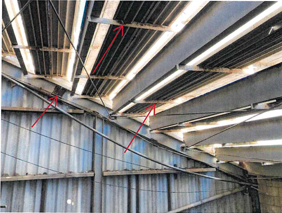
Figure 11 – Photo showing corroded splice plates and cross-members/tread supports (indicated by red arrows)
