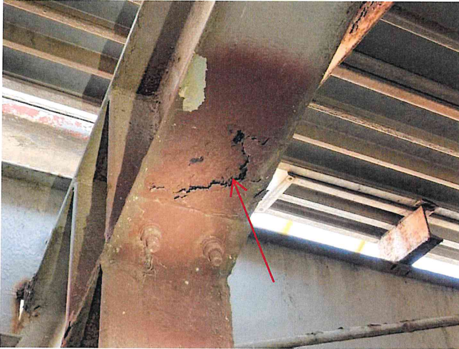
Figure 37 – Photo showing severe corrosion at beam bottom & top flange (indicated by red arrows)
