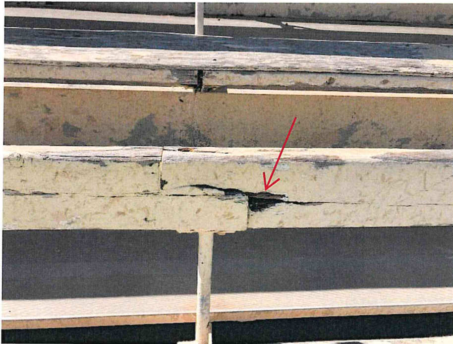
Figure 3 – Close-up photo showing wooden seats and rotted/damaged seat back (note plywood on top of original wood seat)
