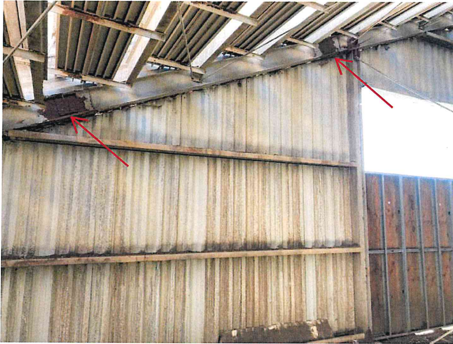
Figure 19 – Photo showing corroded splice plates and cross-members/tread supports (indicated by red arrows)
