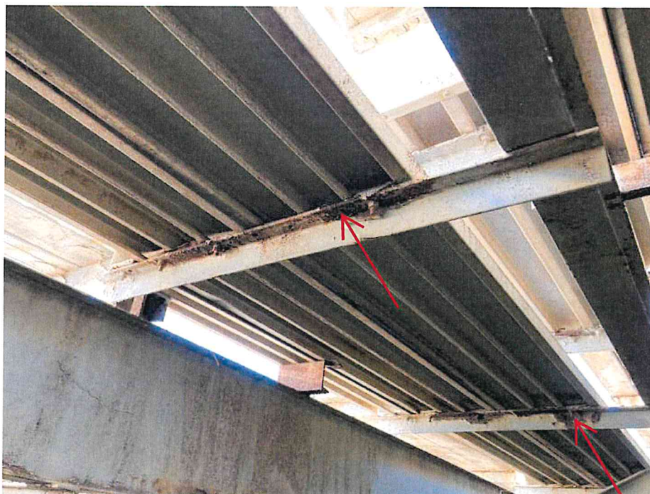
Figure 44 – Photo showing severe corrosion at steel seat support members (indicated by red arrows)
