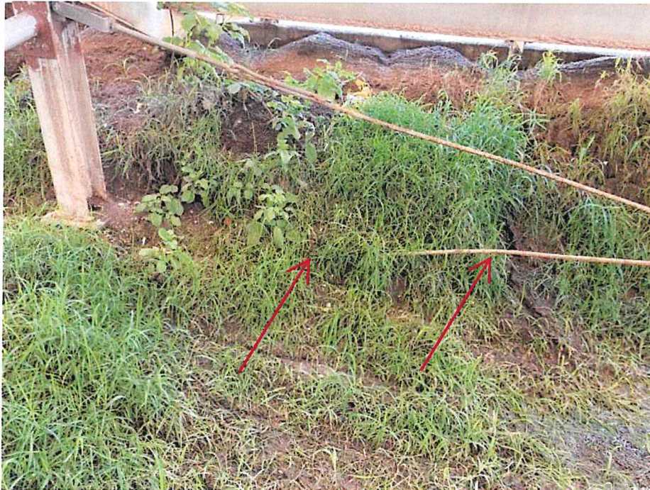
Figure 12 – Photo showing cross-bracing rods bent/damaged and covered by soil
