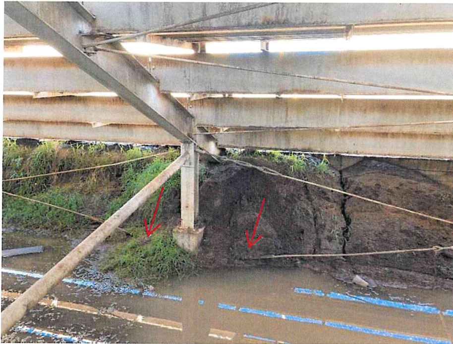
Figure 21 – Photo showing cross-bracing rods bent/damaged and covered by soil
