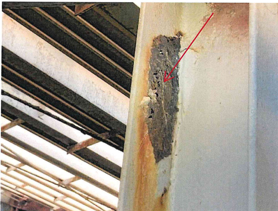
Figure 32 – Photo showing severe corrosion at column flange (indicated by red arrow)
