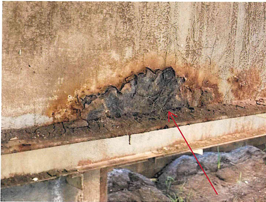
Figure 45 – Photo showing severe corrosion at beam web and flange (indicated by red arrows)
