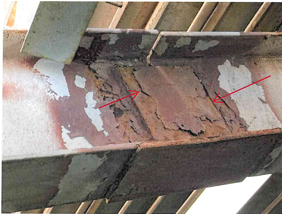
Figure 29 – Photo showing severe corrosion at splice plates (indicated by red arrows)
