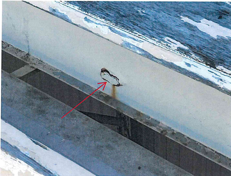
Figure 51 – Photo showing severe corrosion at beam web (indicated by red arrows)
