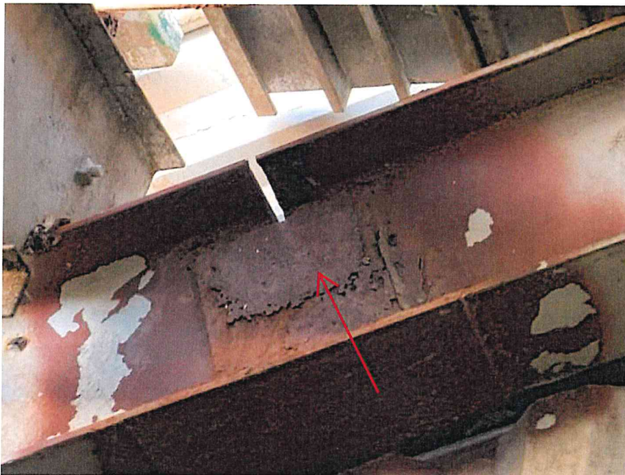
Figure 38 – Photo showing severe corrosion at splice plates (indicated by red arrows)
