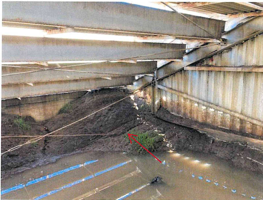
Figure 20 – Photo showing cross-bracing rods bent/damaged and covered by soil
