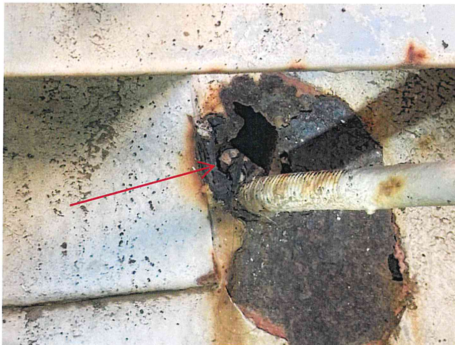
Figure 28 – Photo showing corroded column web at cross-bracing attachment
