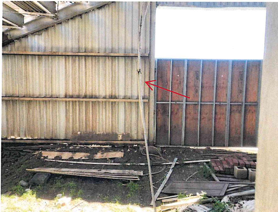
Figure 15 – Close-up photo showing bent/damaged cross-bracing rods
