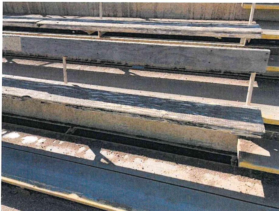
Figure 2 – Close-up photo showing aluminum steps and treads and wooden seats and seat backs (note plywood on top of original wood seat)
