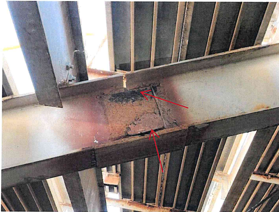
Figure 35 – Photo showing severe corrosion at splice plates (indicated by red arrow)
