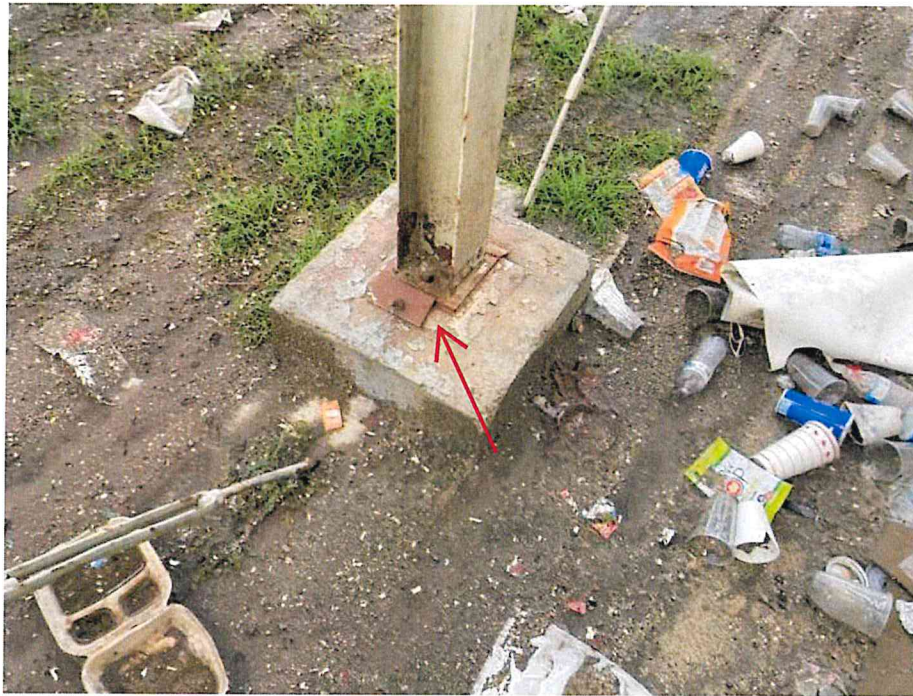
Figure 5 – Photo showing column base with retrofit base plate flanges and anchor bolts
