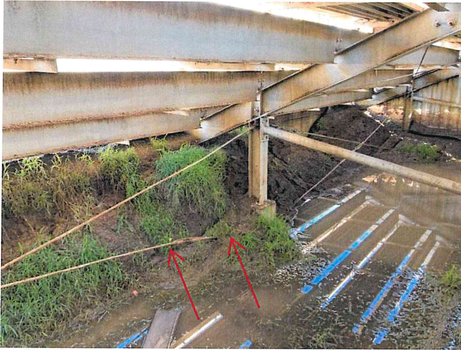
Figure 13 – Close-up photo showing cross-bracing rods bent/damaged and covered by soil
