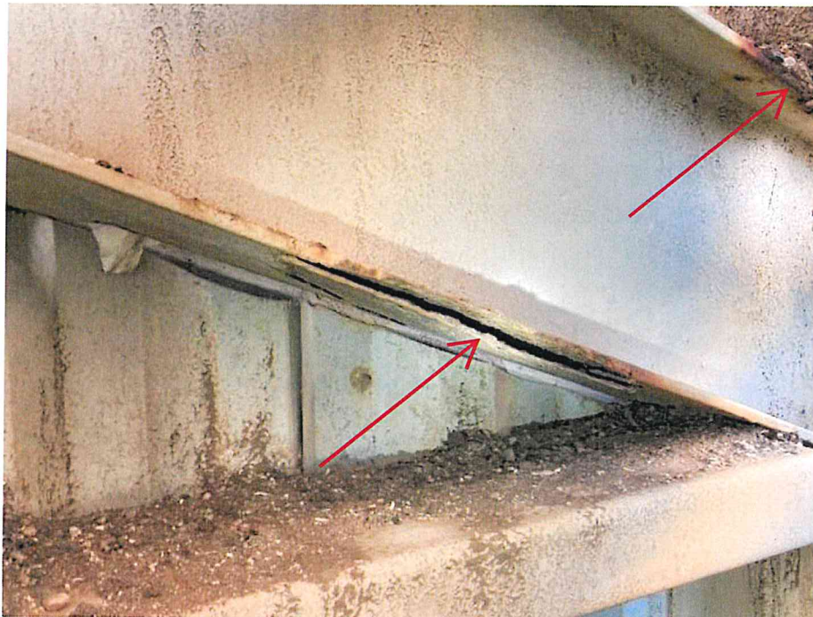
Figure 49 – Photo showing severe corrosion at beam flanges (indicated by red arrows)
